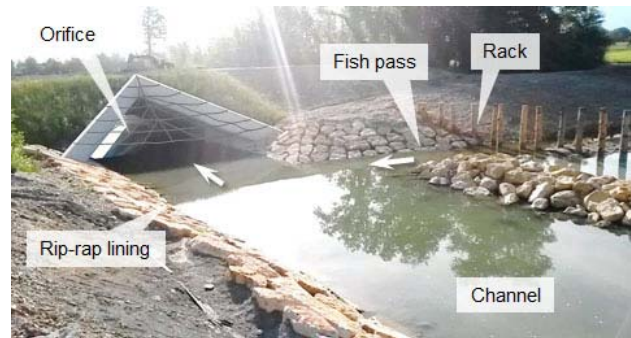
Figure 13: Structures constructed on the Aire River as defined on the physical hydraulic model. A hexagonal orifice and a rip-rap channel bank lining were adopted upstream from the latter.
