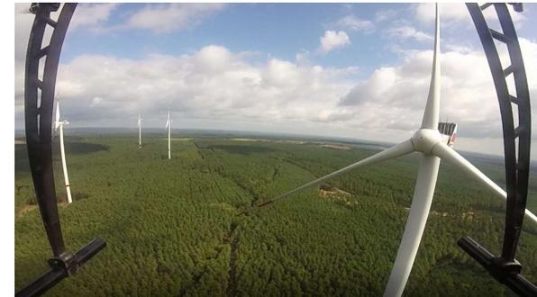
4 WT, in 8 km distance to DVOR, 140 m hub height, 112 m rotor diameter
