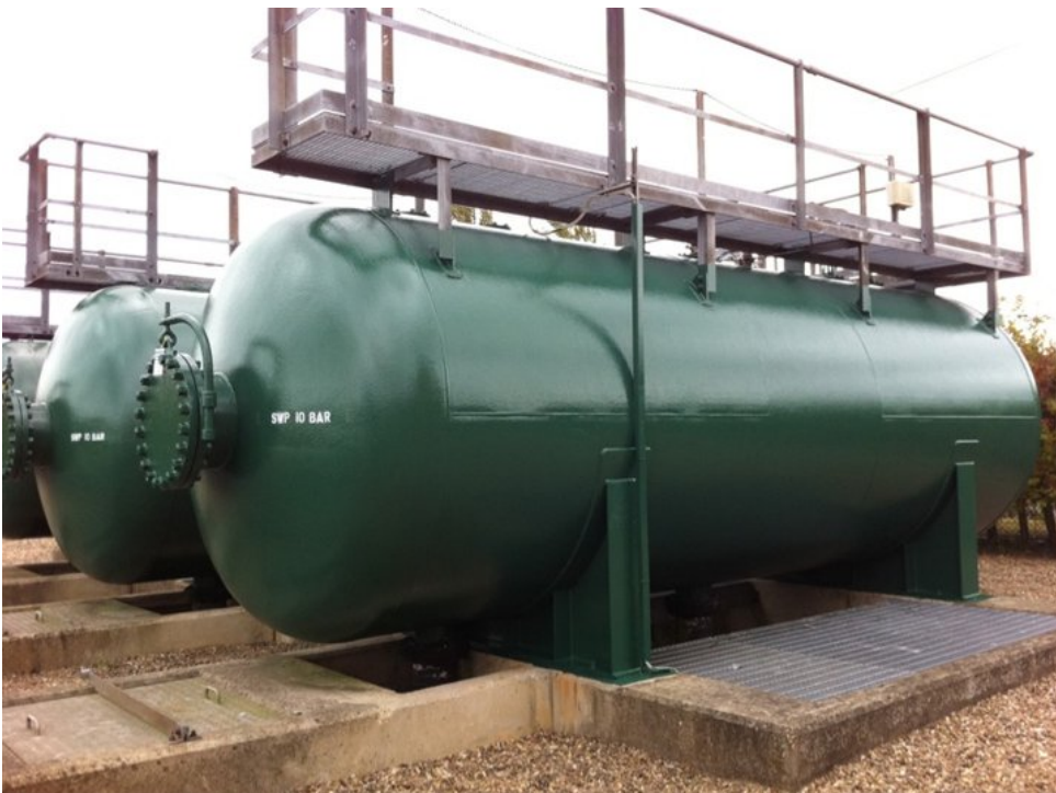
Figure 3.8 Example of horizontal surge tanks in Amman. Provided by Miyahuna (M. Abualshaikh), 2025.
