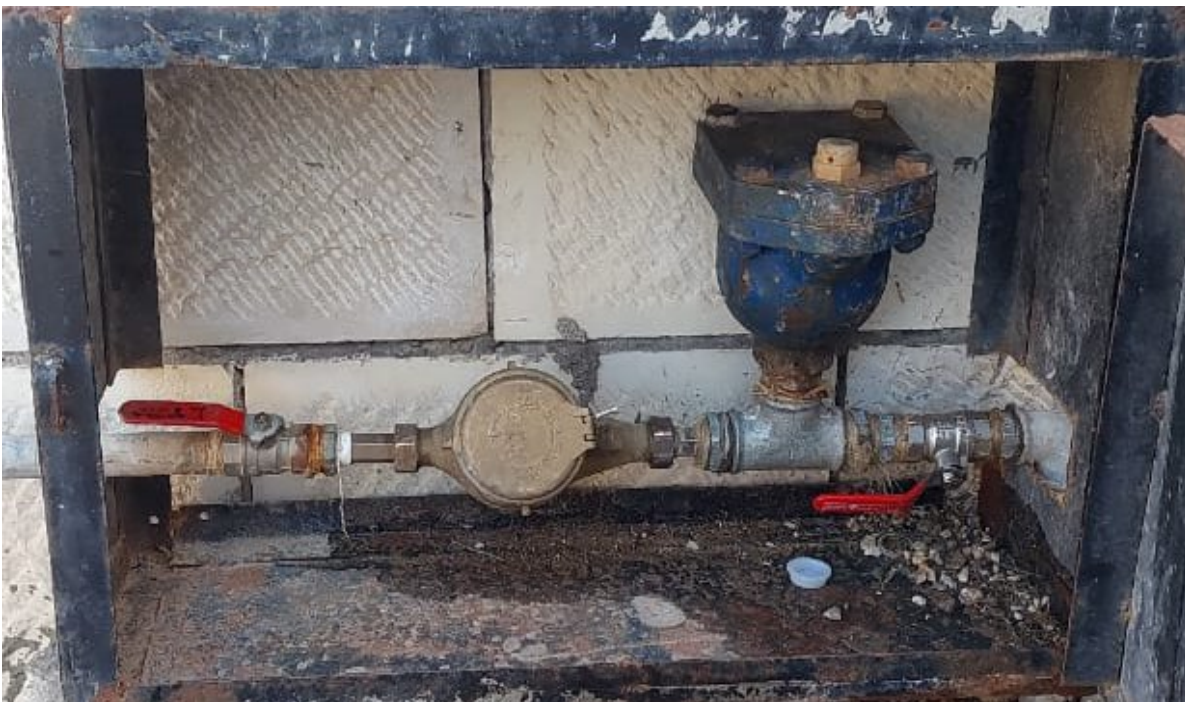
Figure 3.2 Installation of a domestic air release valve. Image provided by Miyahuna (M. Abu-alshaikh), 2024.
