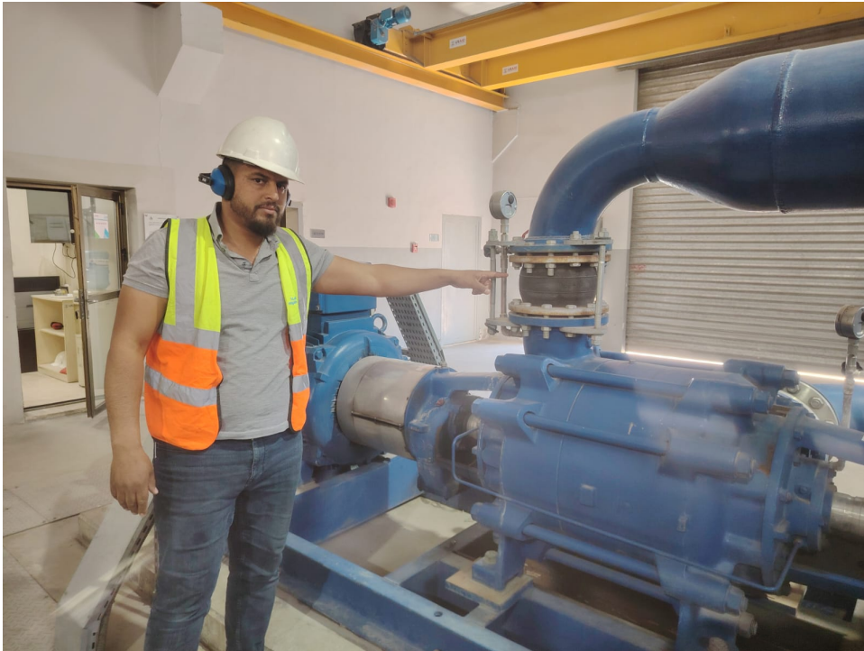
Figure 3.7 Example of flexible piping attached to a pump. This installation reduces the stress on the pipes. Image provided by Miyahuna (M. Abualshaikh), Amman, 2025.
