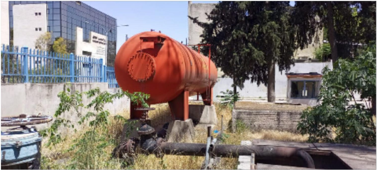
Figure 3.5 Horizontal surge tank in Amman, image provided by Miyahuna (M. Abualshaikh), 2025.
