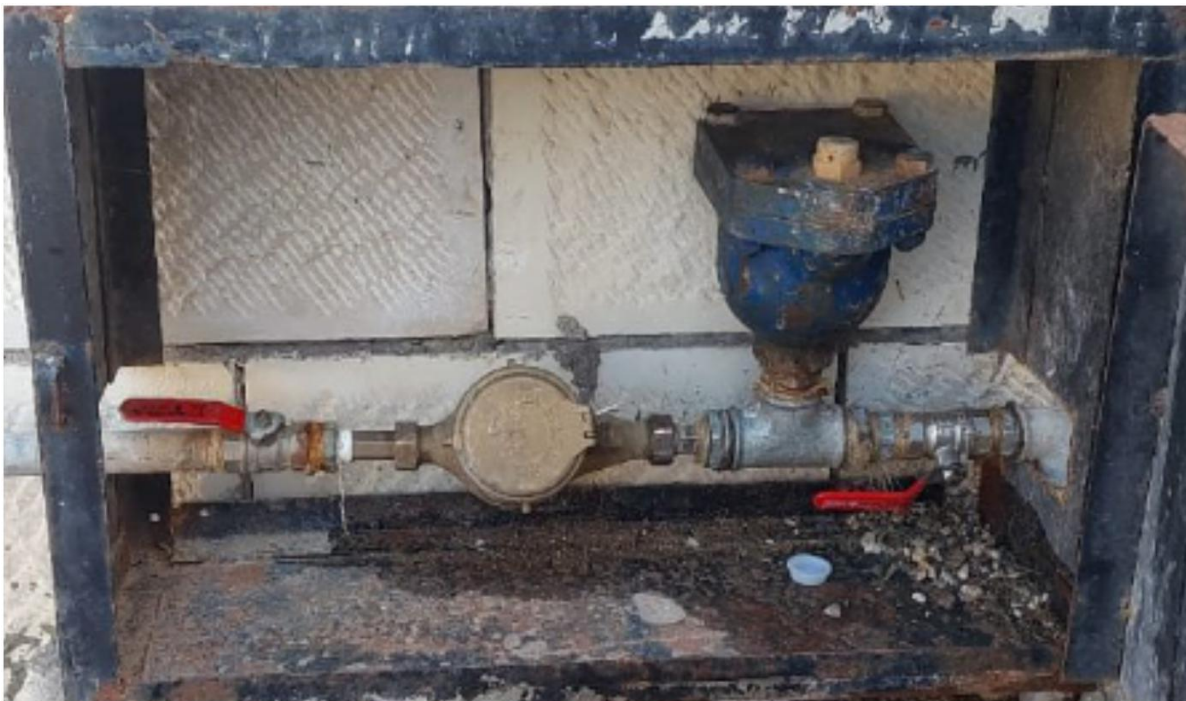
Figure 3.2 Installation of a domestic air release valve. Image provided by Miyahuna (M. Abu-alshaikh), 2024.
